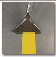
Begin LeanStripe removal with a scraper. Getting under the LeanStripe with the scraper, peel up 1-2 inches (2-5 cm) of striping.
